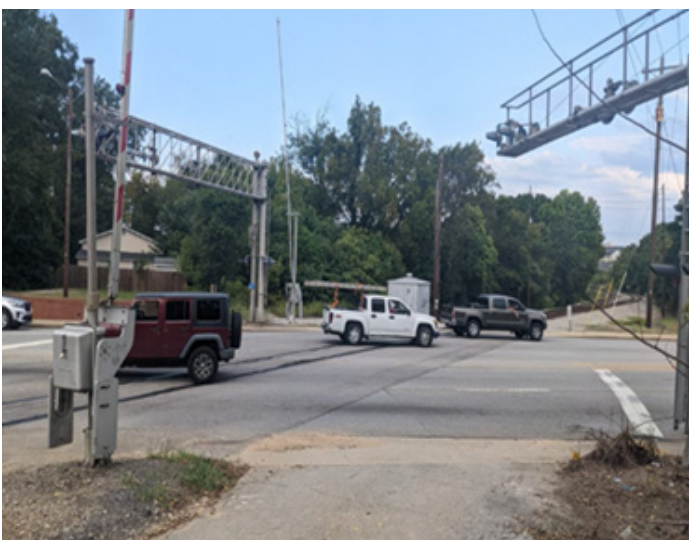
Huger Street Crossing
