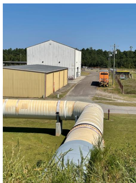
Vent piping with warehouses added later in the background
