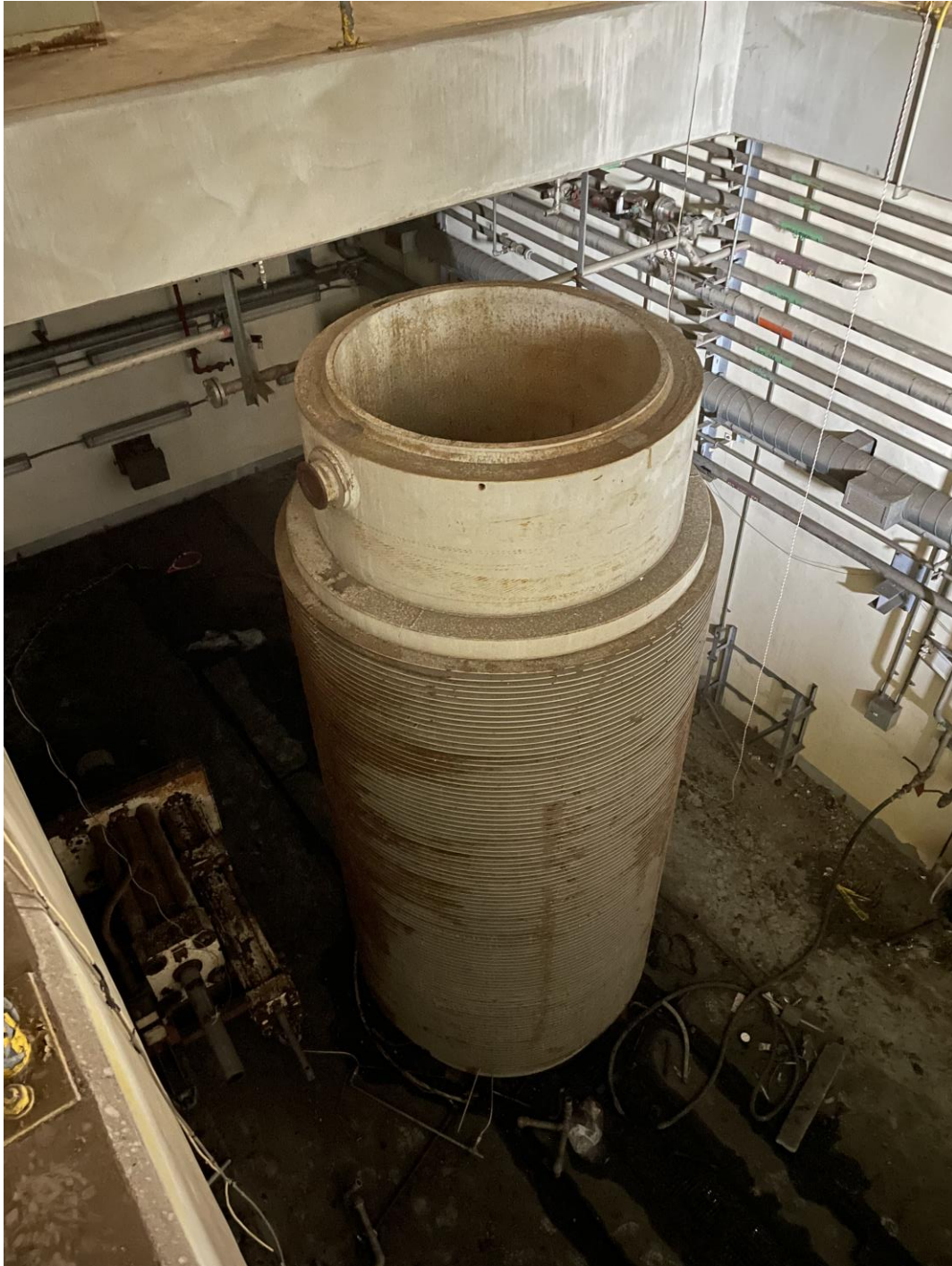
Steel training cask for fuel rod transport
