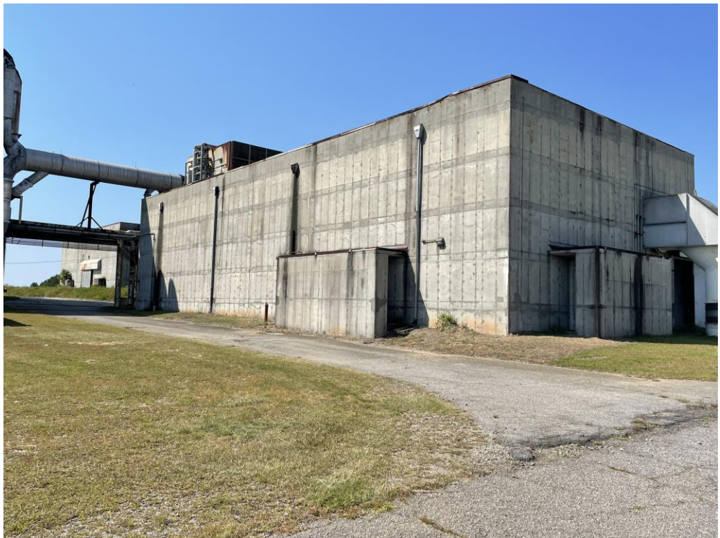
Ventilation fan, filter and ductwork building
