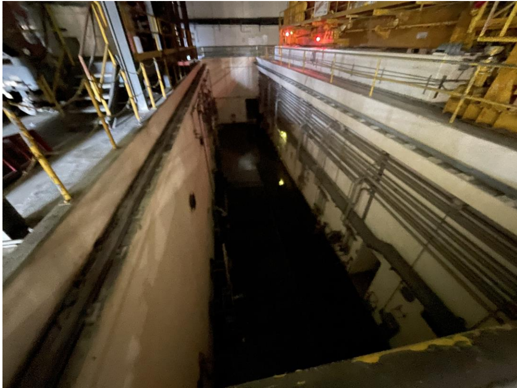
Cask wash pit
