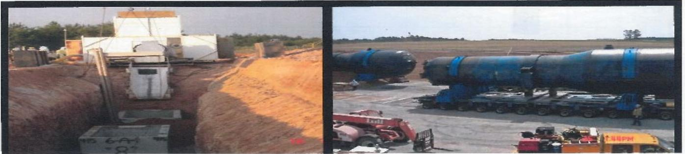
Large components, irradiated hardware, are also part of the operation that we do there, and the picture you see two steam generators that were buried at Barnwell. These are the components that the 13 reactors that are currently part of the compact that we are trying to provide to space for, for disposal.
